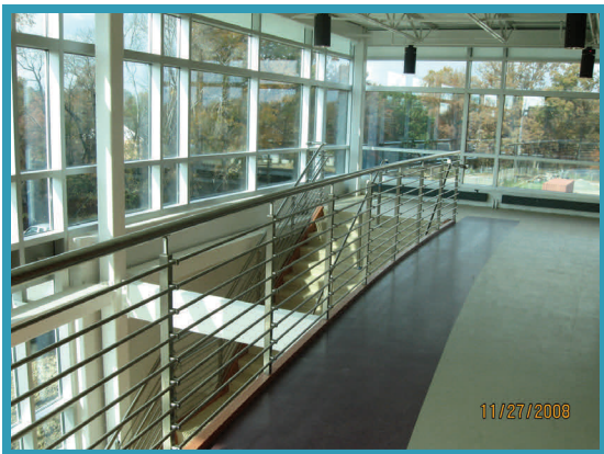
Cable Railing Job
